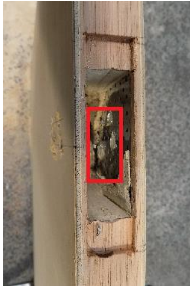
Modified Internal of the Door Leaf – Extra core section removal shown in Red.
